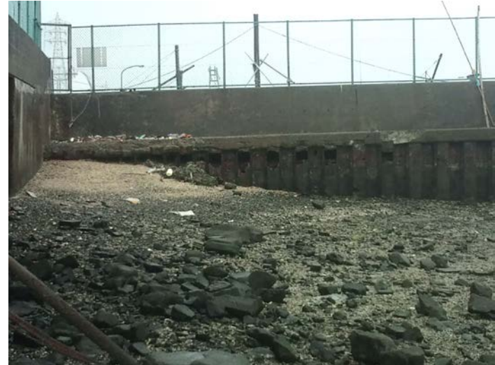
②西防波堤
